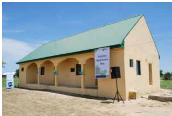
The construction of the History Economic Centre, Umar Suleiman College of Education, Gashua executed by Yobe Branch
