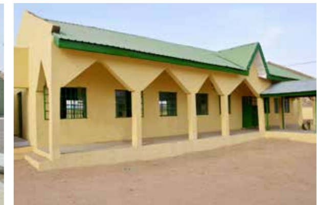
The renovated Shagari Health Care Centre Gusau by Our Northwest 2 Regional Bank
